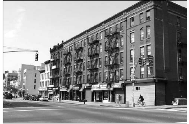
West side of Second Avenue, view south from 119th Street 2
