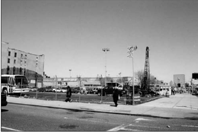
West side of Second Avenue, view north from 126th Street 1
