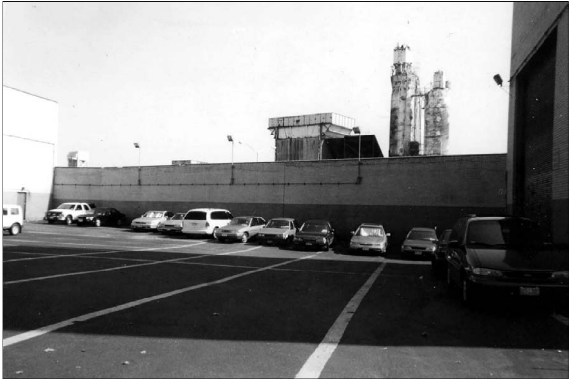
Site A - Looking north at Site A from 128th Street
