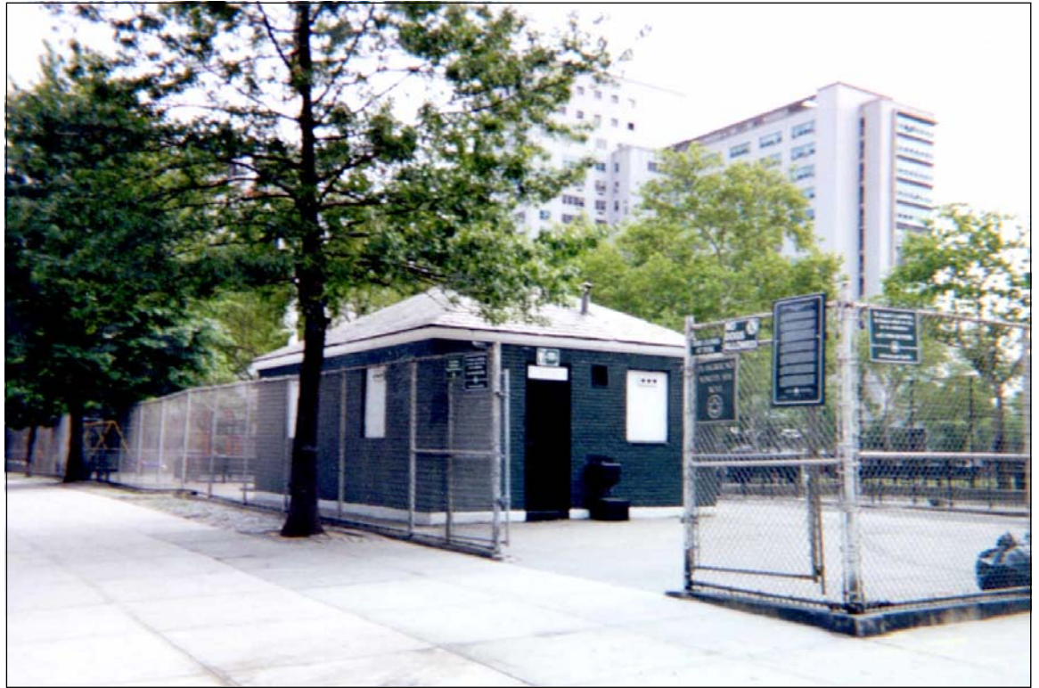
Site D - Looking northeast at site from Second Avenue and 96th Street
