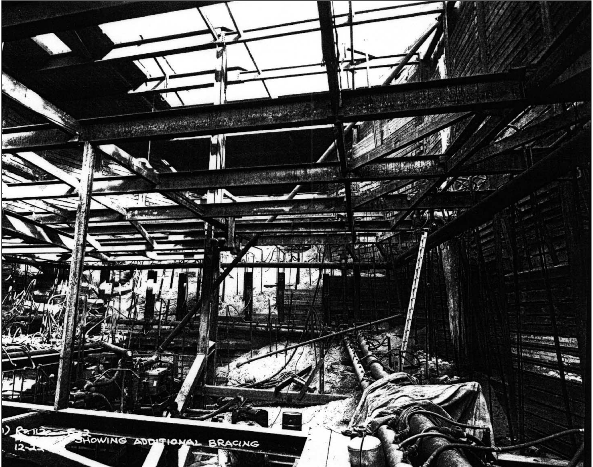
Photograph showing construction of subway beneath Chrystie Street with temporary steel piles that were left in place after completion of the tunnel
