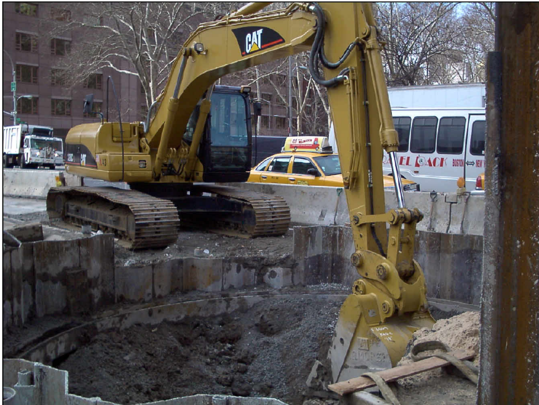
Steel sheeting and bracing
