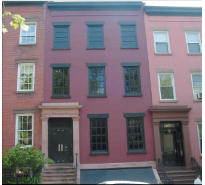
Example of existing ancillary vent facility in Brooklyn
