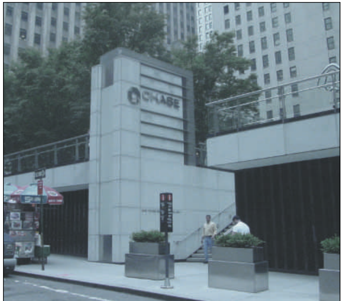
Example of existing ancillary vent facility in Manhattan
