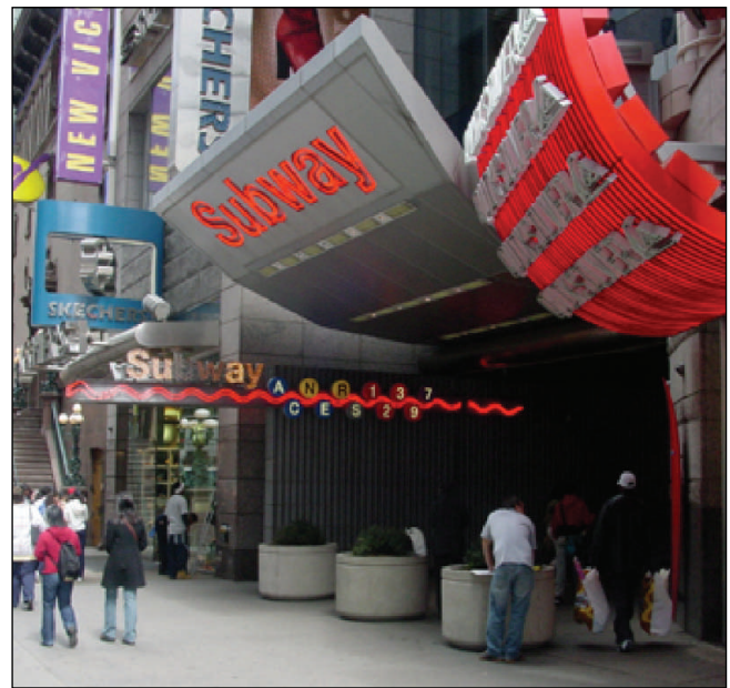
Illustration of an existing off-street entrance to the subway system
