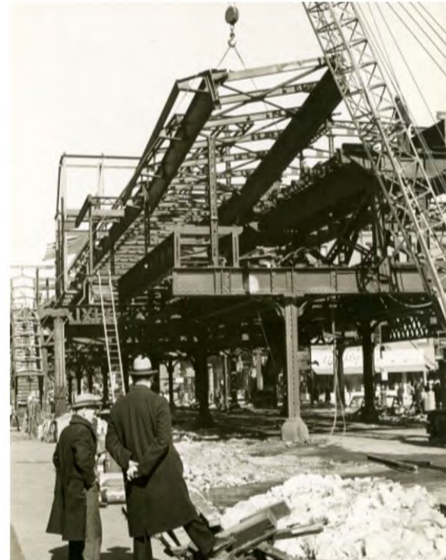
Dismantling of Second Ave. Elevated Line in the 1940's
