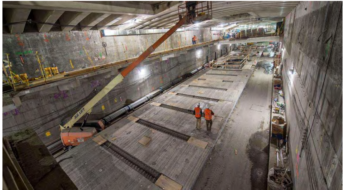
Manhattan – Terminal Pre-Cast Platform and Mezzanine Levels in April 2018
