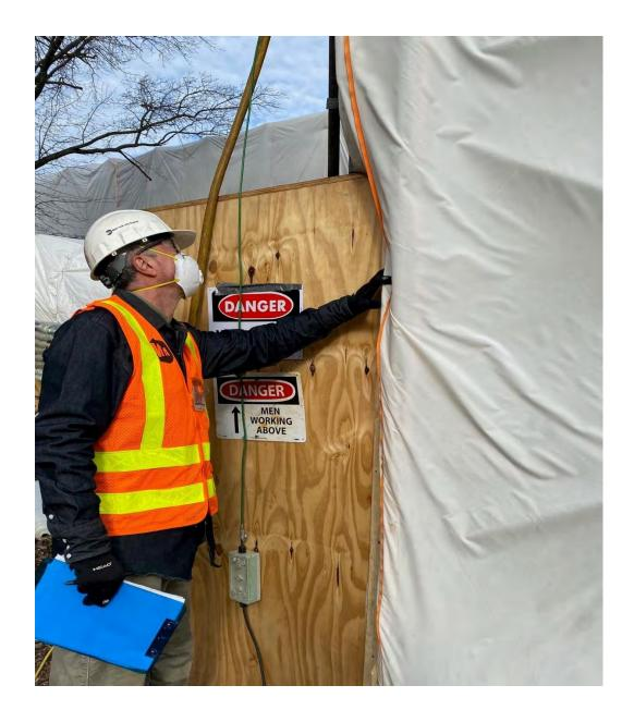
Recent photo of System Safety Specialist, Oscar Suarez, from the Office of System Safety, as he inspects the active abrasive blast operation containment system at the 180th Street Station restoration project on the 2/5 Line in the Bronx.
