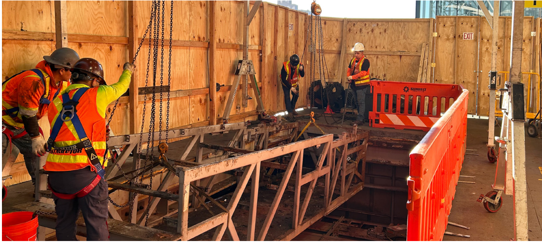
Crews prepare to remove the out-of-service moving walkway at Jamaica Station
