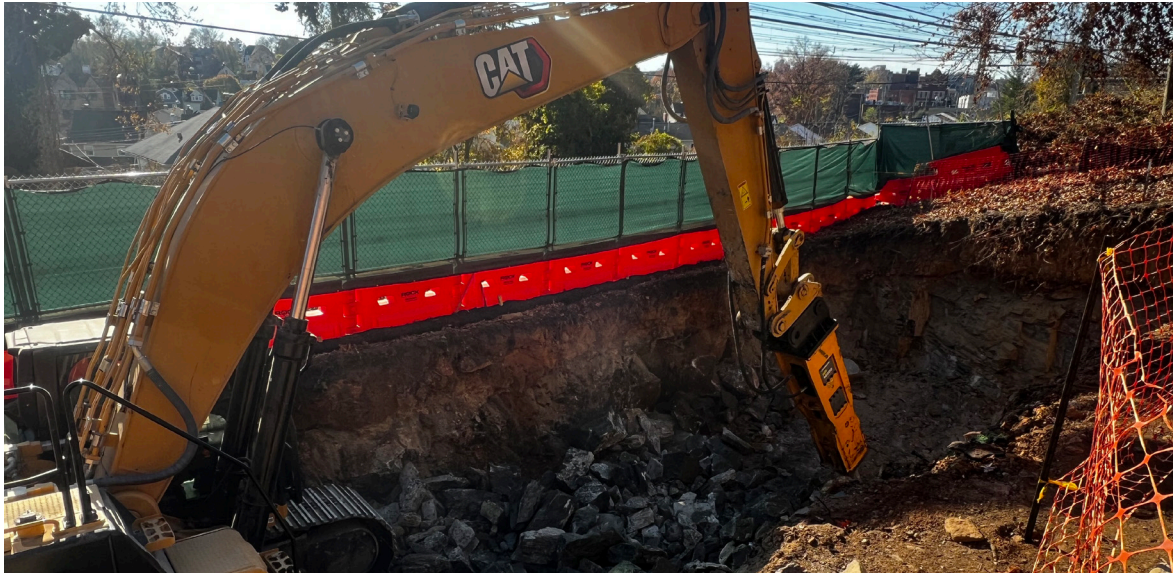
Crews replace the Pelham Substation on the New Haven Line
