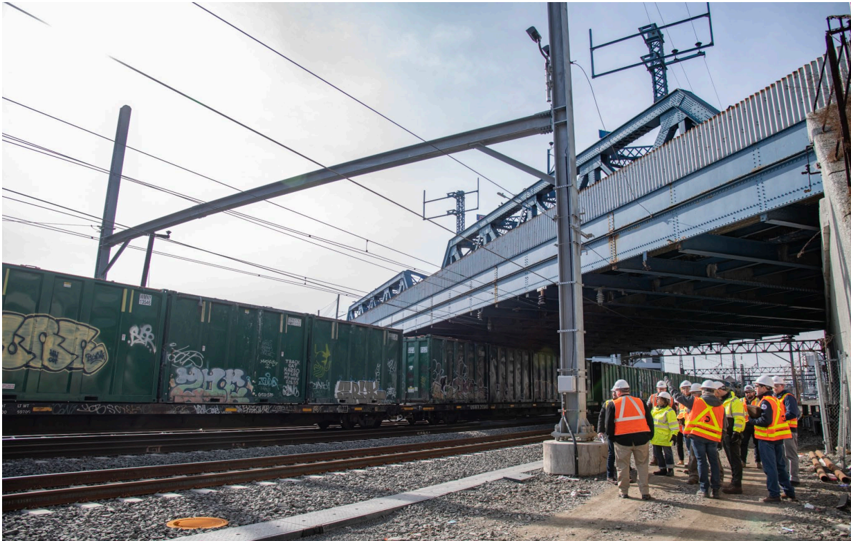
Completed portal near Leggett Interlocking, February 2024
