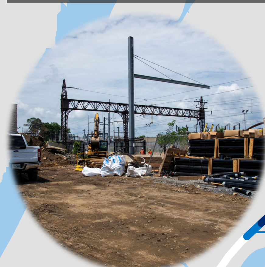
New and old catenary structures near Parkchester/Van Nest Station, August 2024
