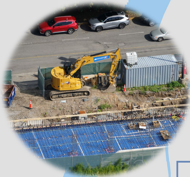
Foundation underway at HG Substation, November 2023
