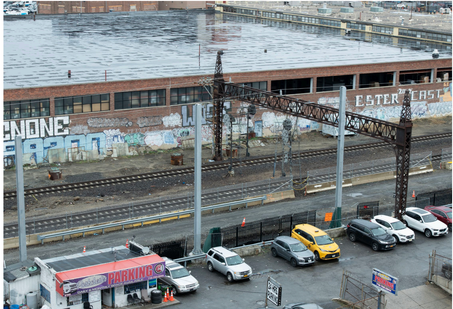
Original portal and new columns near Parkchester/Van Nest Station Site, February 2024
