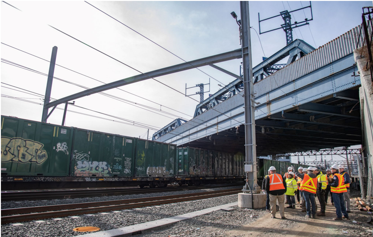
Completed portal near Leggett Interlocking, February 2024
