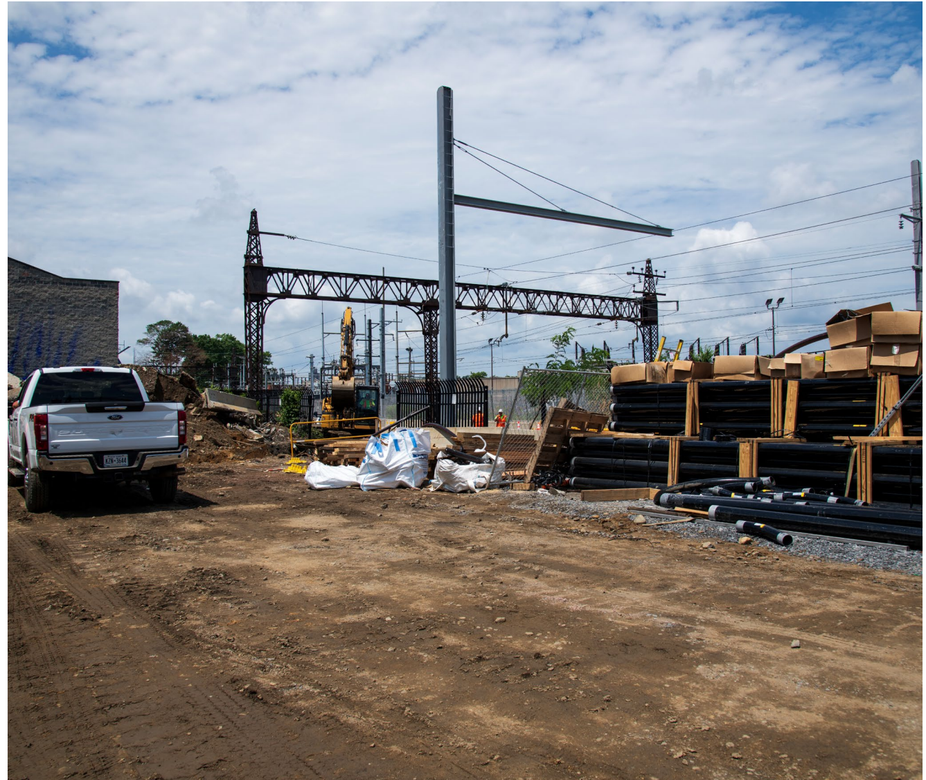
New and existing OCS portals installed near Parkchester/Van Nest Station, July 2024
