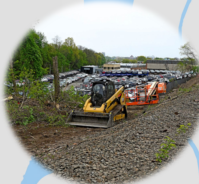
Site preparations underway at HG2 Substation, April 2024
