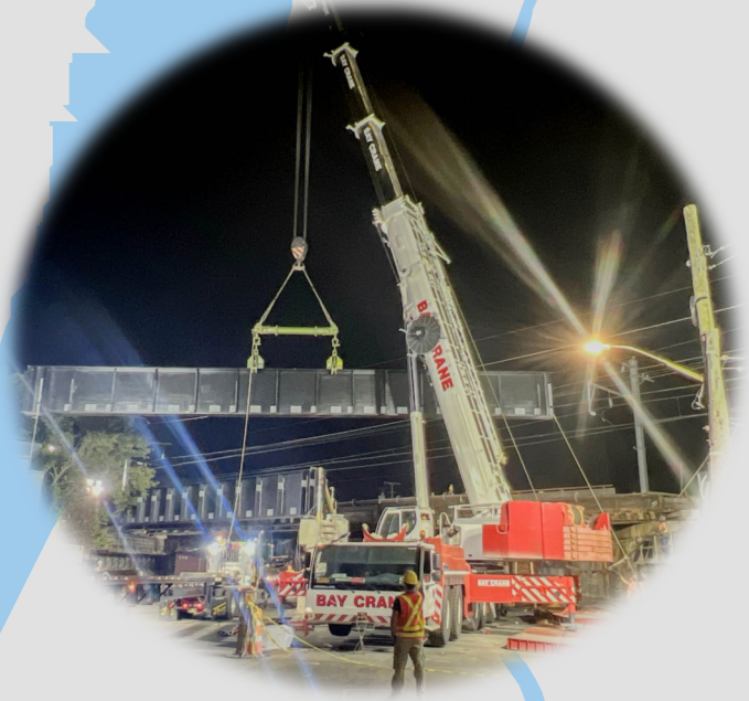
Crews complete new steel installation at Bronxdale Ave Bridge, August 2024
