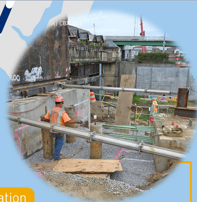
Footing installation at Hunts Point Station site, August 2024
