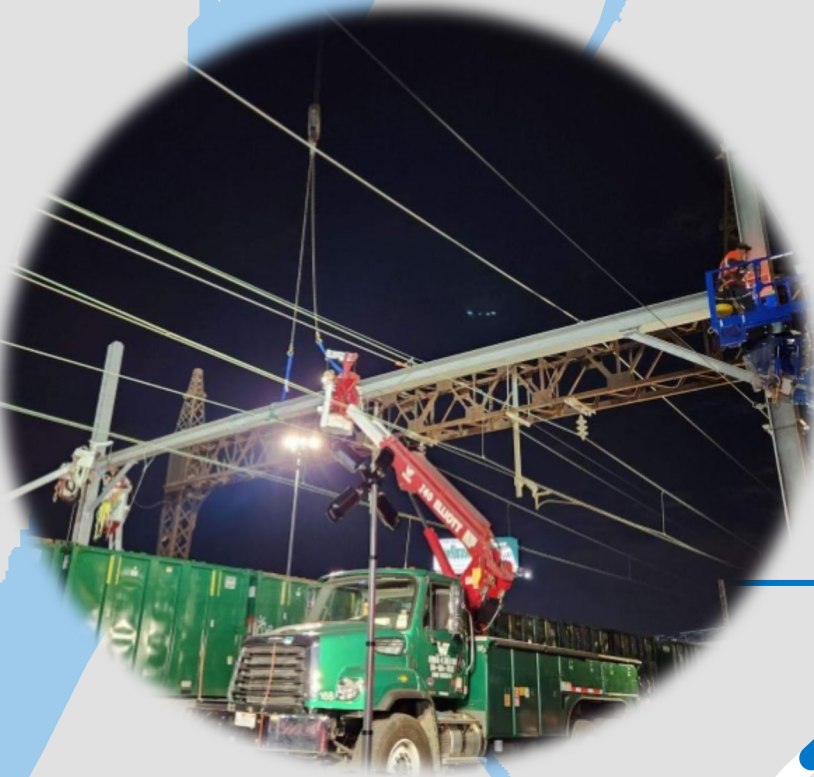
OCS portal installation near Leggett Interlocking, October 2023
