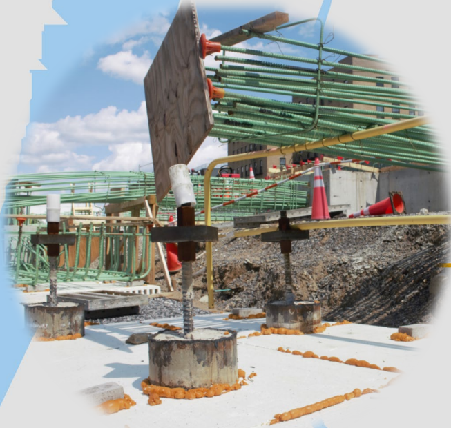
Micropiles, rebar, and concrete installed at Hunts Point Station site, August 2024
