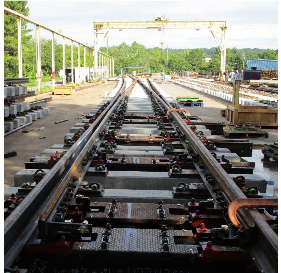
Factory test of fabricated railroad crossovers and switches at Voestalpine Railway Systems Nortrak facility in Birmingham, Alabama, August 2022
