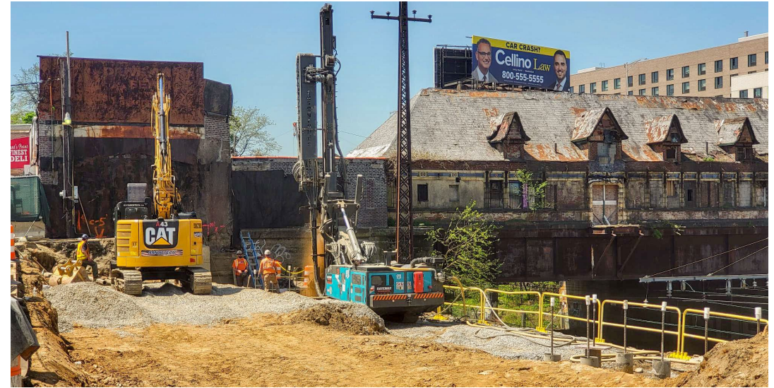
Crews drill micropiles at Hunts Point Station site north entrance, May 2024
