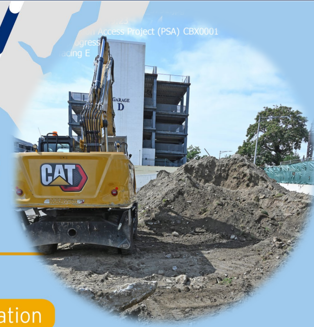
Site preparations at Morris Park Station Site, August 2024
