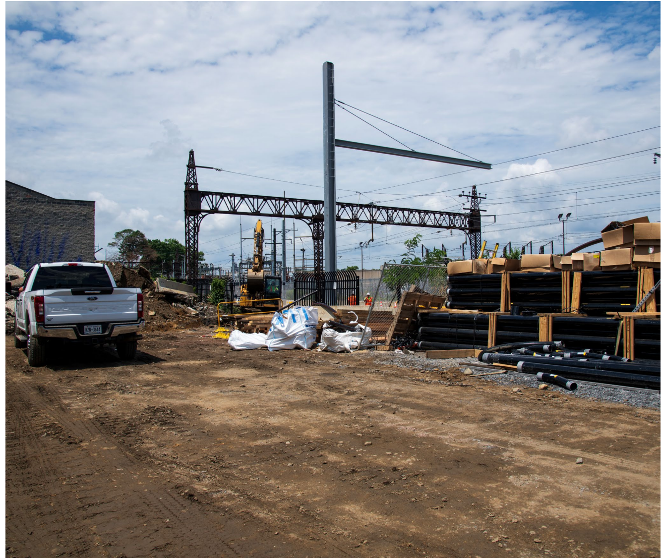
New and existing portals at Parkchester/Van Nest Station, July 2024
