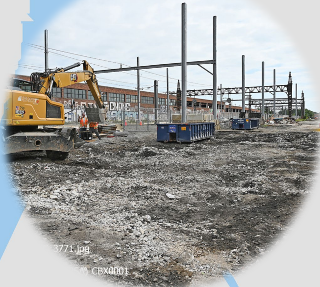
Site preparations at Parkchester/ Van Nest Station Site, August 2024
