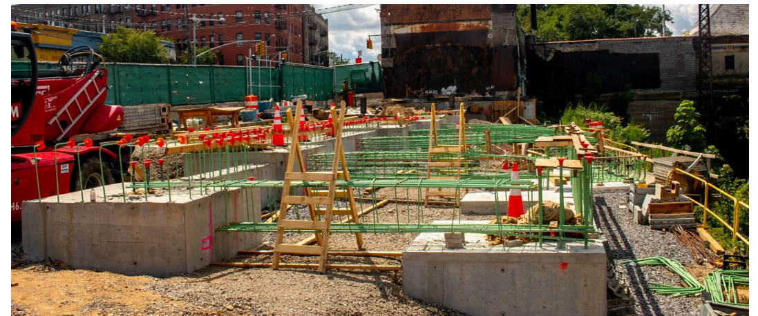
Installed concrete and rebar at Hunts Point north entrance, August 2024
