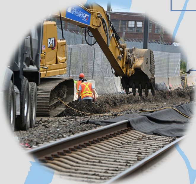
Site preparations underway near Van Nest Substation, July 2024
