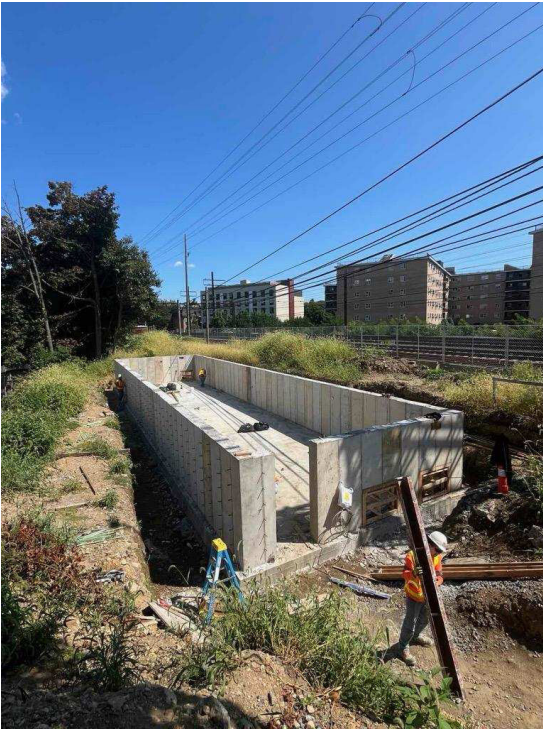
Crews are reconstructing two substations on the New Haven Line.
