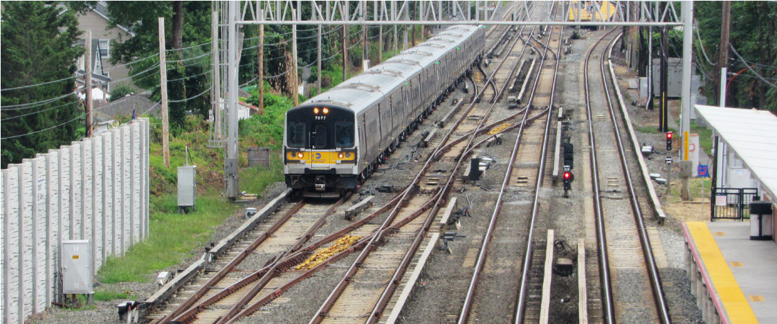
Crossovers and signals on LIRR tracks
