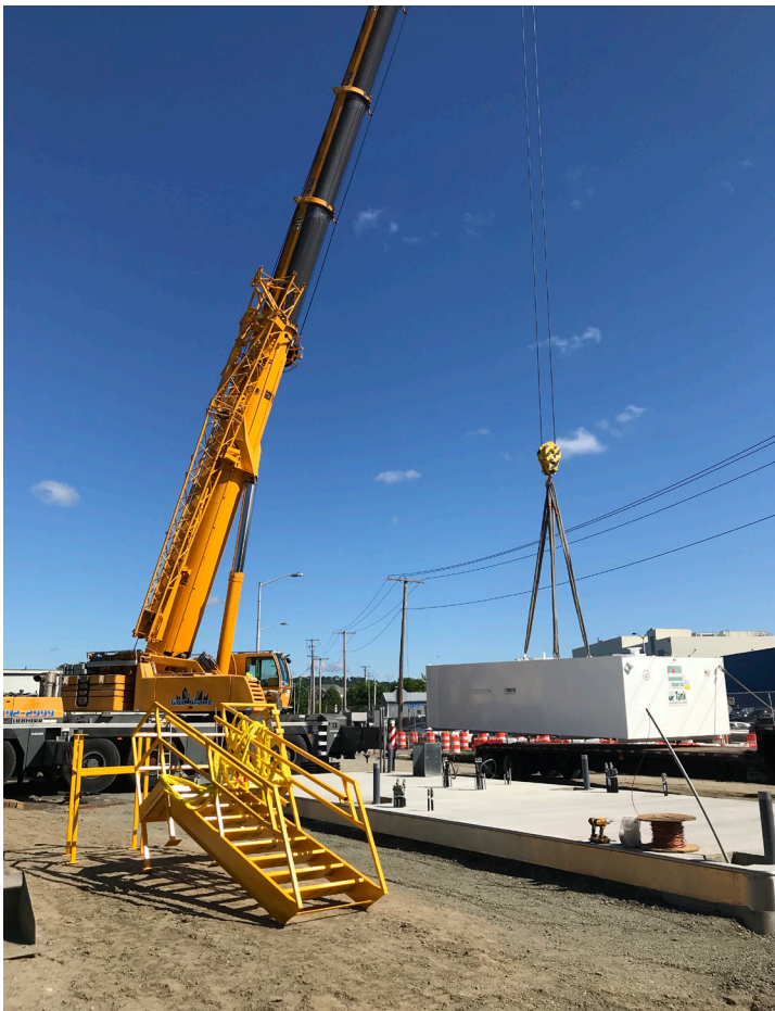
Crews work to replace Underground Storage Tanks to support Metro-North operations
