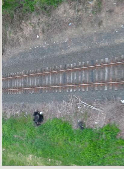
DEBRIS ALONG THE RIGHT OF WAY
