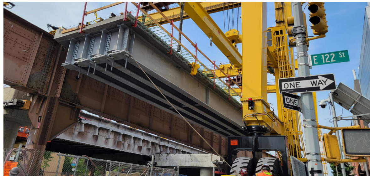
Crews work to replace the aging Park Avenue Viaduct
