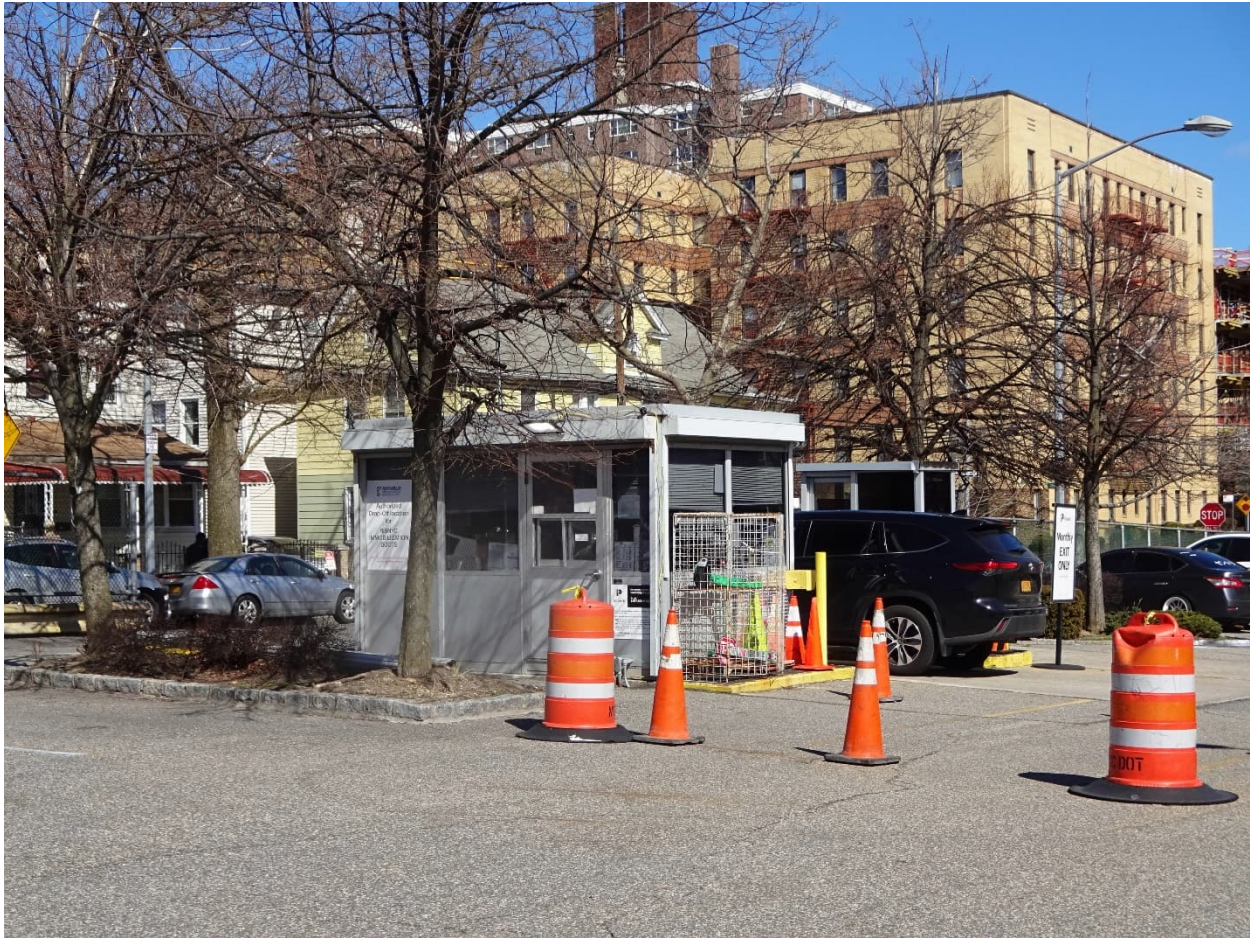
Figure 4.2-3: Existing Ticketing Booth to Be Removed
