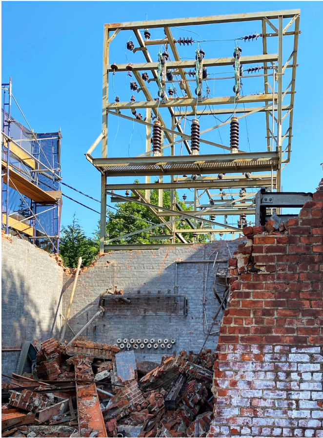
Demolition of the Hempstead Substation
