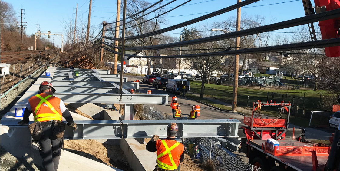
Crews prepare the area around Babylon Interlocking for signal system modernization.
