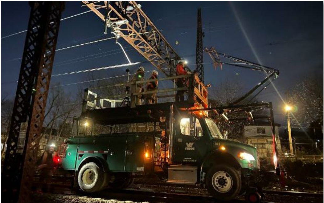
Plate C Overhead Catenary Structure (OCS) Wire Raise Inspection
