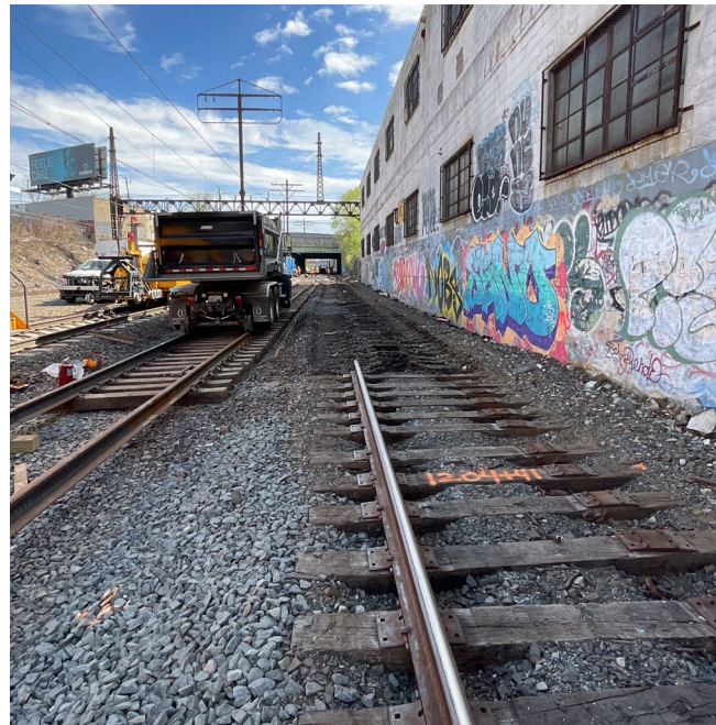
Demolition of Track 5
