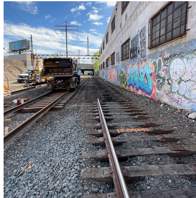
Demolition of Track 5
