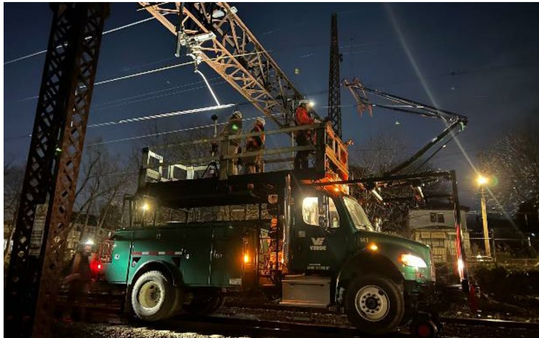
Plate C Overhead Catenary Structure (OCS) Wire Raise Inspection
