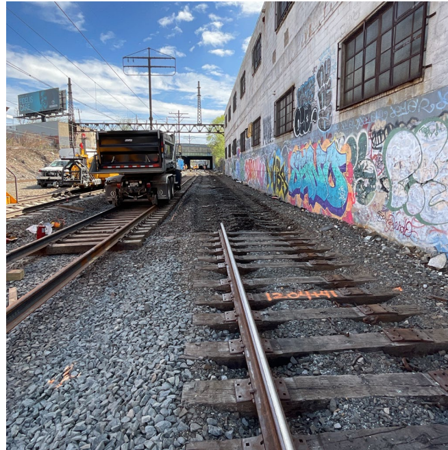
Demolition of Track 5
