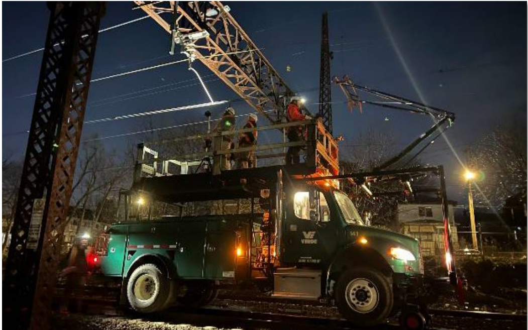
Plate C Overhead Catenary Structure (OCS) Wire Raise Inspection
