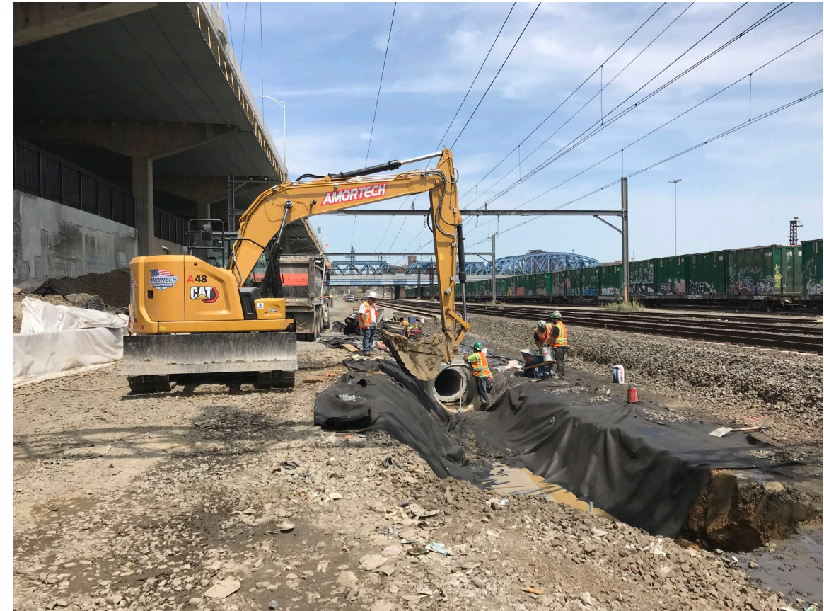
Drainage system installation near Leggett Interlocking
