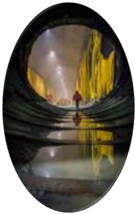
8 miles of new tunnels and 40 miles of new track
