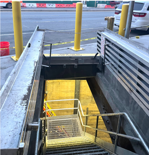
An open hatchway under street level used for access and emergency egress.
