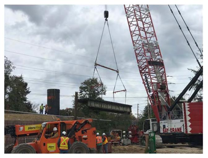
**Acabonac Road Bridge Replacement:** An alternative service plan went into effect in October to support the replacement of two (2) LIRR Bridges over North Main Street and Accabonac Road in East Hampton. The replacement bridges will increase the elevation of the tracks to lower the chance of bridge strikes in the future. Service restoration is planned for November 10, 2019.
