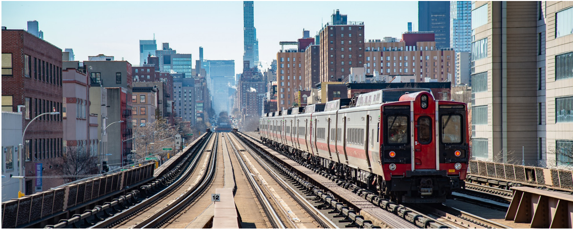
A Metro-North train traverses the over 100-year-old Park Avenue Viaduct in Manhattan.
