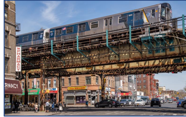
NYCT Elevated Structures Enhanced Overcoating Program
