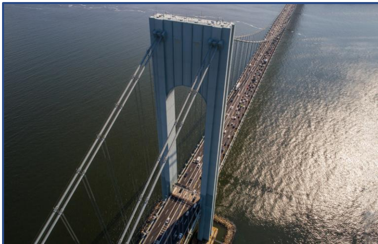
B&T Verrazzano Narrows Bridge Main Cable Dehumidification
