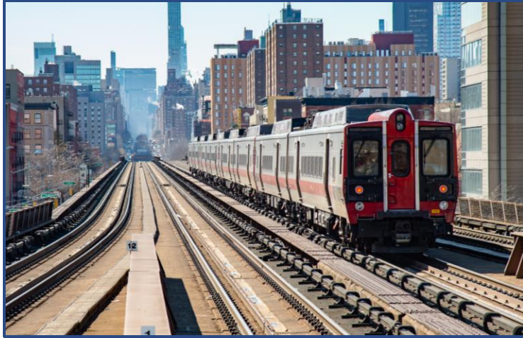
Metro-North Park Avenue Viaduct Phase 2 Acceleration
