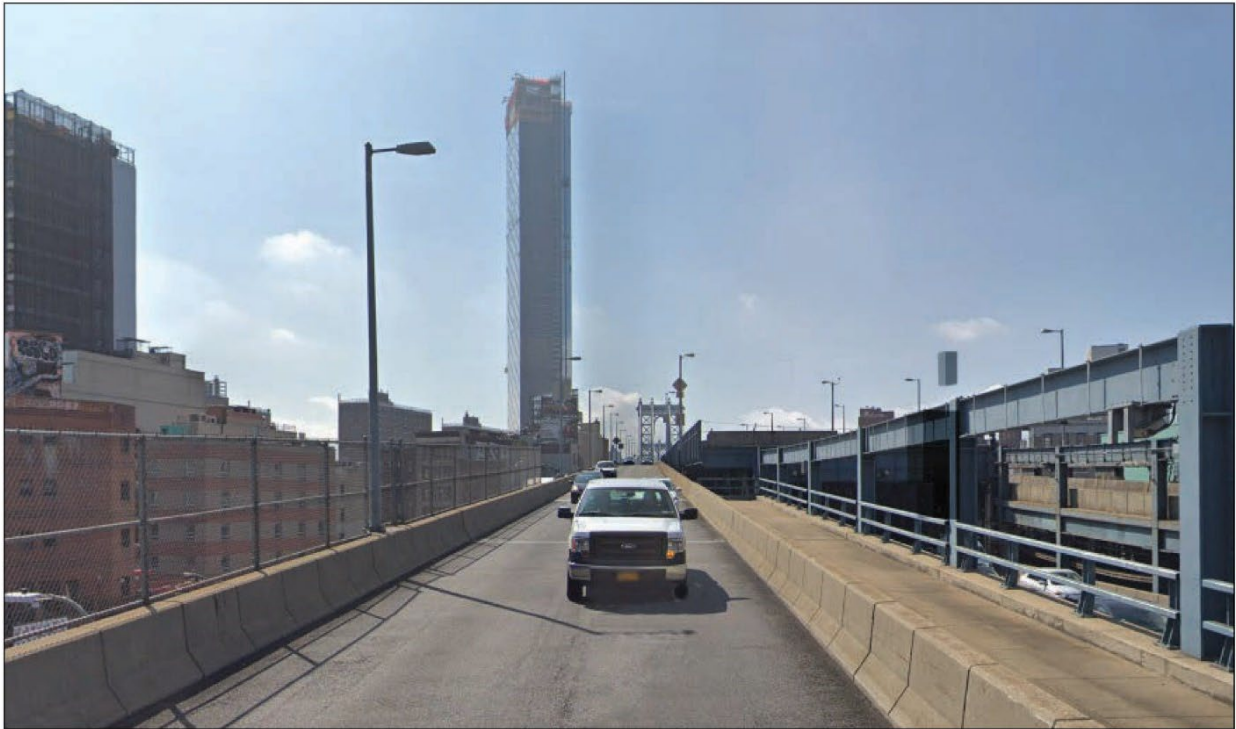
No Action Alternative, view southeast
