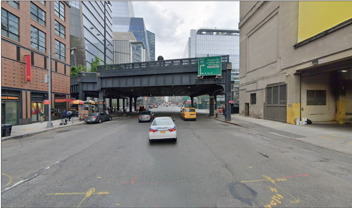
No Action Alternative, view north on Tenth Avenue
