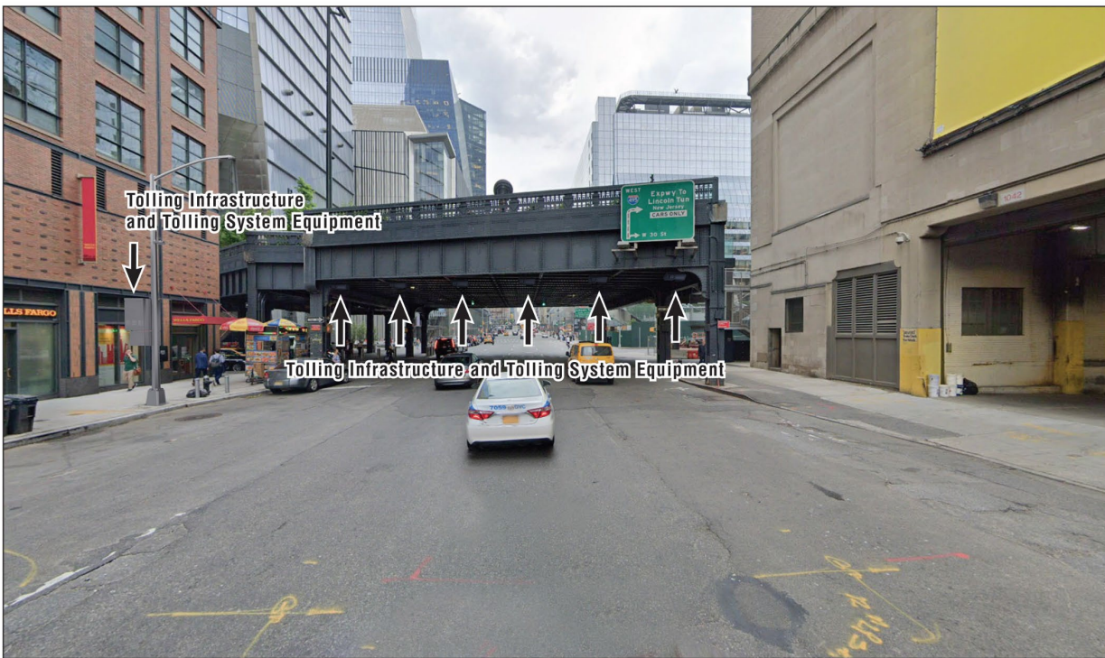
CBD Tolling Alternative, view north on Tenth Avenue
