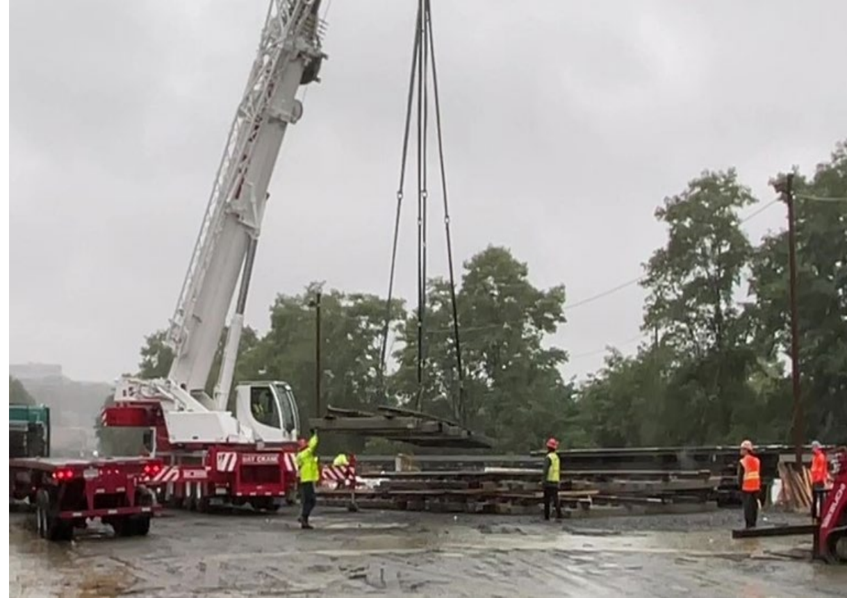
Delivery of Leggett Crossover special track work
