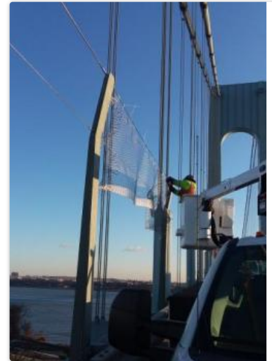
Installation of fencing on the Verrazzano-Narrows Bridge
