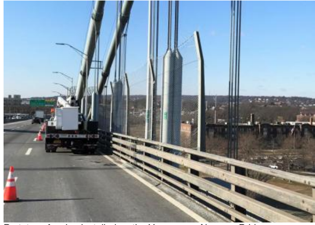
Prototype fencing installed on the Verrazzano-Narrows Bridge.
