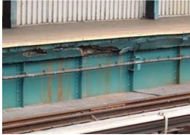
Examples of girder deterioration at 111 St.
