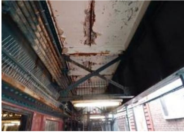
Examples of girder deterioration at 111 St.
