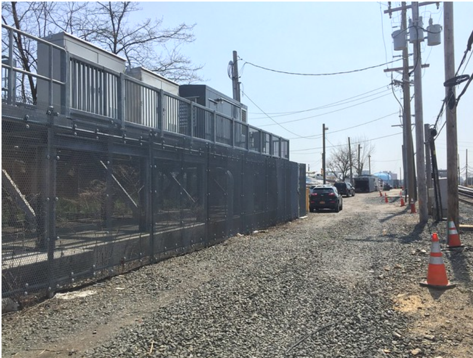
LIRR's Long Beach Branch signal, power and communications are being fully replaced and elevated above flood levels or hardened in place with flood-resistant materials and techniques.
