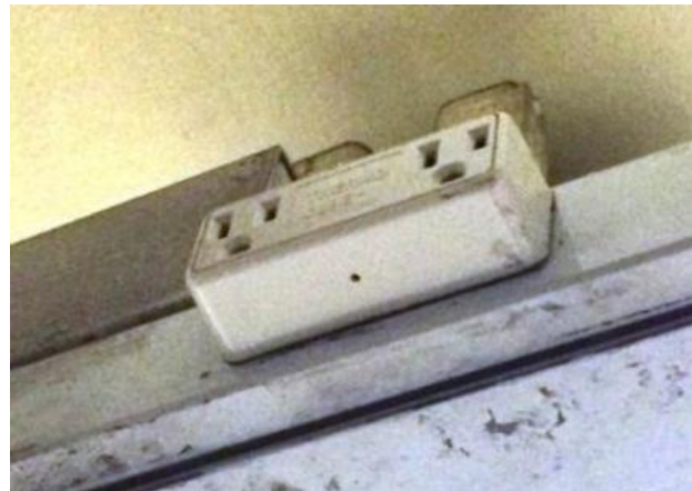
Pin hole at bottom of plug adapter mounted to cable channel located above MVM (contains camera)
