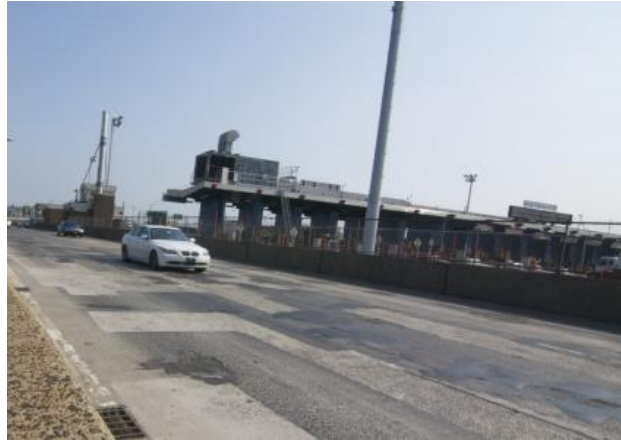
Example of a section of the RFK Bridge's Manhattan/Queens ramp showing multiple roadway patches. The RFK Bronx toll plaza is to the right. The fenced area is where the temporary bridge roadway was constructed.
