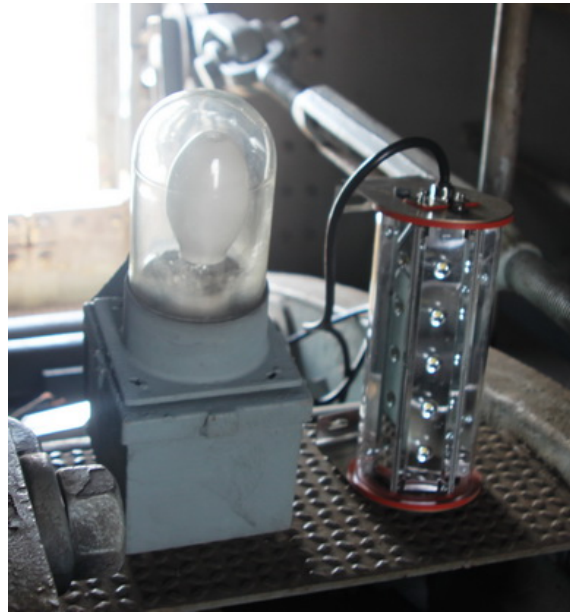
LED2: (left) old mercury vapor light; (right) new, energy-efficient LED light
