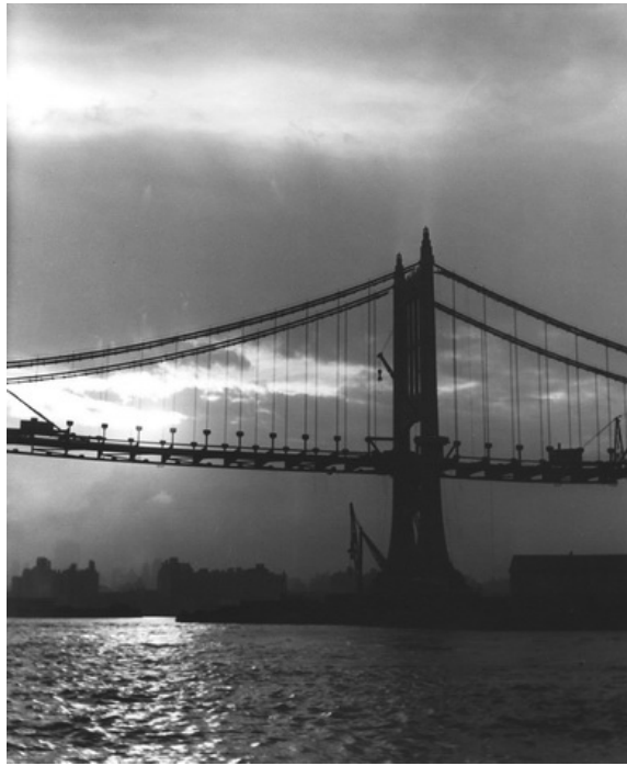
Triborough Bridge_Suspended Span: Getting ready to put in the roadbed at the Triborough Bridge's suspended span. 1935. Photographer unknown.
