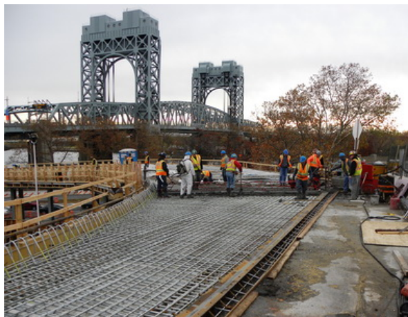
HRD Ramp1: New rebar put in place before concrete deck is poured on the new Harlem River Drive ramp to the RFK Bridge. The Harlem River Lift Span is in the background.
