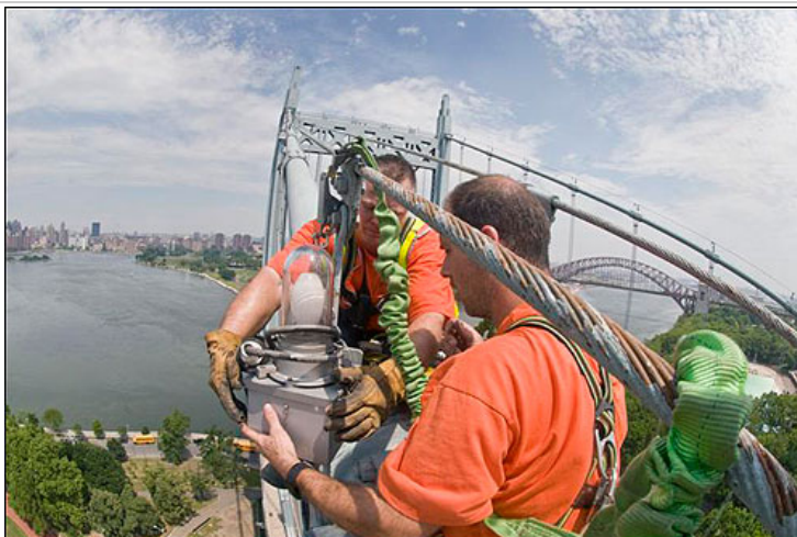
Bridge and Tunnel Maintainers Charlie Torrillo (foreground) and Jeff Calichio (facing front) remove old mercury necklace light from atop the Robert F. Kennedy Bridge.
