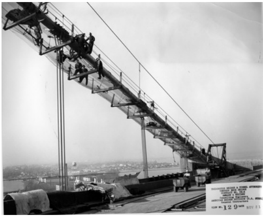
Wrapping west cable on Bronx side of bridge. Nov. 21, 1960. Mal Gurian Associates.
