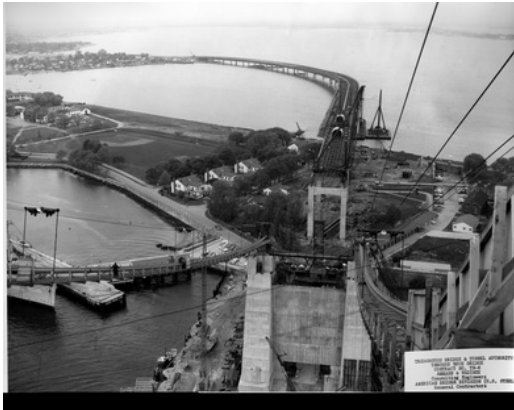
View of Bronx side span looking north from Bronx tower. Spinning of the 9th set-up on the west cable is in progress. May 16, 1960. Mal Gurian Associates.
