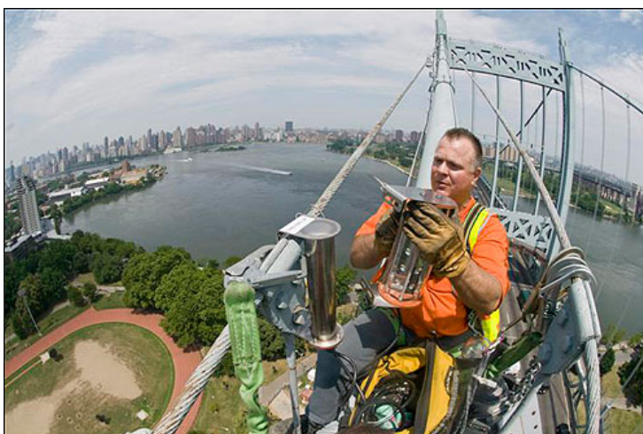
B&T Maintainer Jeff Calichio installs new energy-efficient LED light atop RFK Bridge. LED lights help cut the amount of electricity needed to power the necklace lights by 73 percent.
