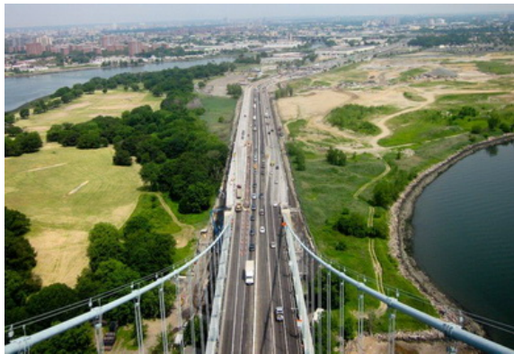
Bronx Approach showing newly constructed breakdown shoulders, viewed from top of the Bronx Tower looking north. (Photo credit: Jeff Brugge for MTA Bridges and Tunnels.)
