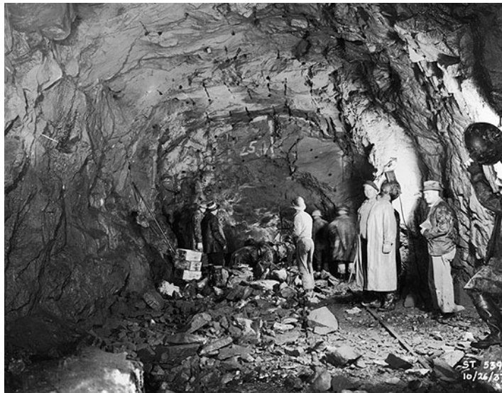
Photo 3: South tunnel bottom drift, west of Queens construction shaft. Oct. 26, 1937. Rappaport Studios. Courtesy of MTA Bridges and Tunnels Special Archive
