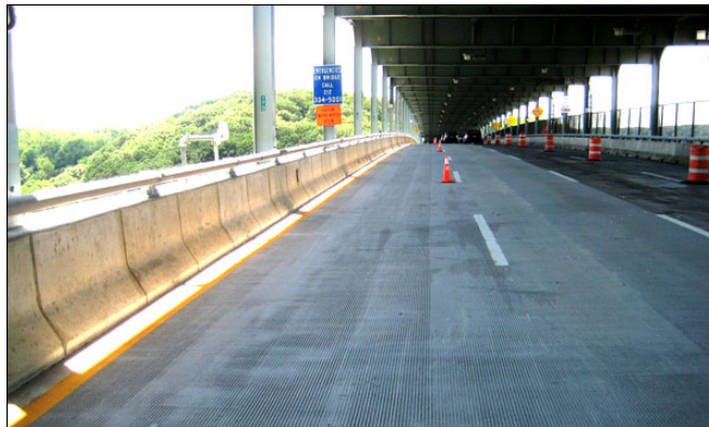
(After) Brand new deck replaced the bridge's original 1930's-era roadway.
