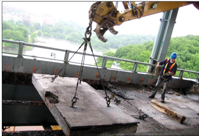
(Before) Concrete slab is removed from roadway during construction work at Henry Hudson Bridge.
