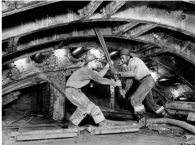
Photo1: Sandhogs tighten a bolt in a tunnel–lining ring. Six cylindrical jacks on the back of a shield are visible behind the men. Photographer: Michael Bobco for Somach Photo Service. Feb. 26, 1939. Courtesy of MTA Bridges and Tunnels Special Archive
