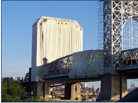
Tower of RFK Bridge's Harlem Lift Span under environmental containment for paint removal.
