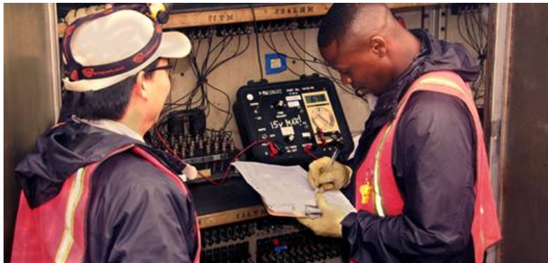
Signal men performing functional tests following fire at Hall Tower.
