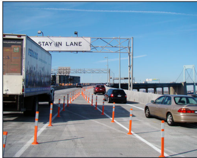
One-lane configuration on Cross Island Parkway northbound ramp to Throgs Neck Bridge provides motorists with a dedicated lane and no merges.
