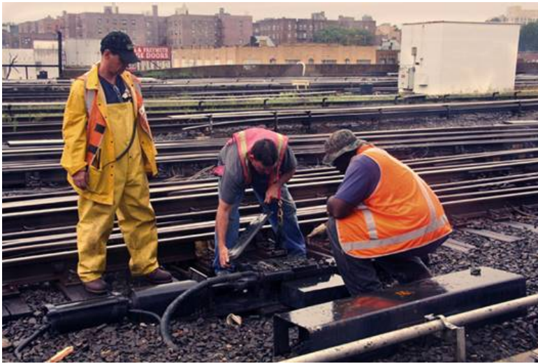
Signal men checking control wires within a switch machine.
