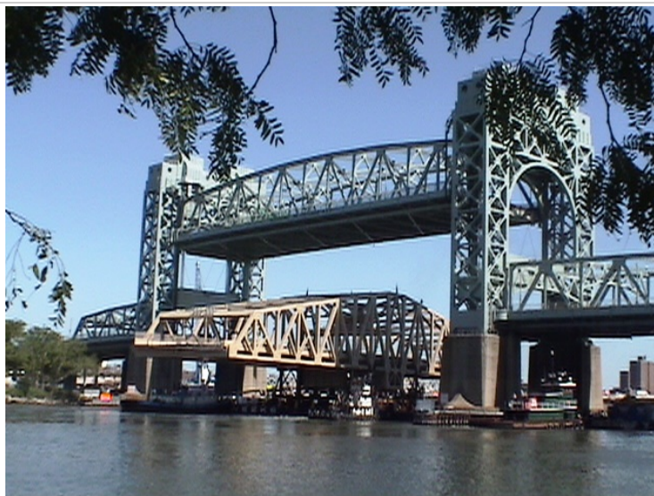
NYC DOT's new Willis Avenue Bridge as it travels beneath Robert F. Kennedy Bridge's Harlem River Lift en route to its final home. (Photo credit MTA Bridges and Tunnels/Raymond Bush.)
