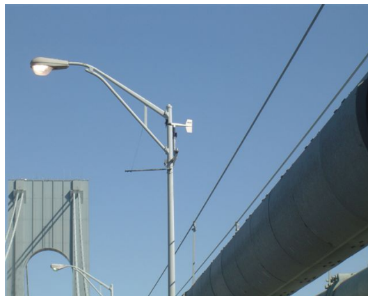
View of weather sensor inconspicuously attached to light pole at the Verrazano-Narrows Bridge.
