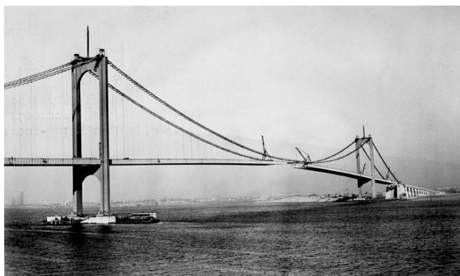
Bronx-Whitestone Bridge under construction
