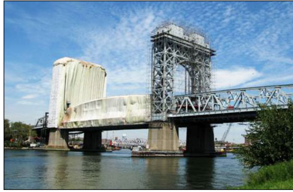
PHOTO CAPTION: Sections of Triborough Bridge's Harlem Lift Span shrouded for environmentally contained paint job.
