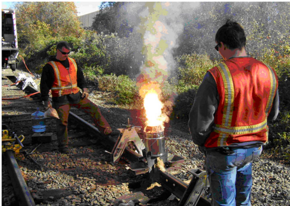
Welding of rail joint in process
