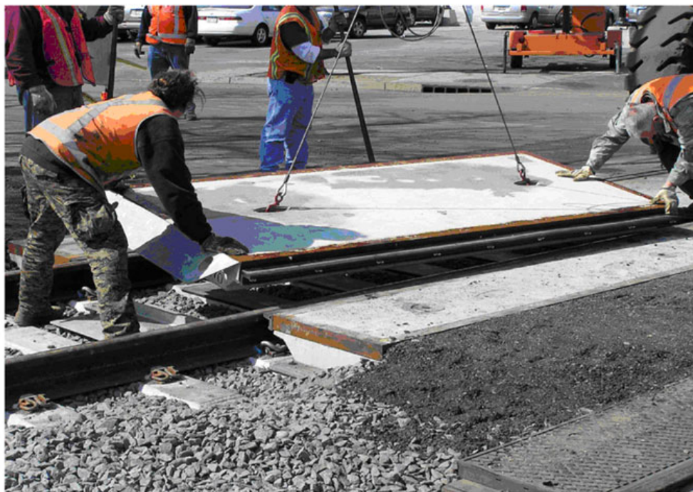
Installation of concrete crossing panel
