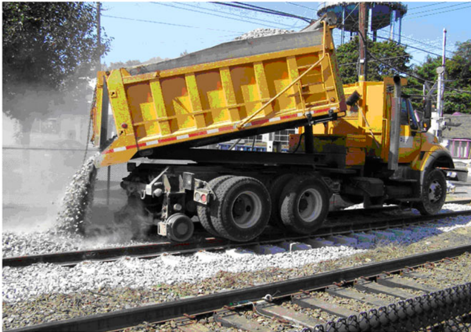
Stone ballast being dumped in preparation of surfacing
