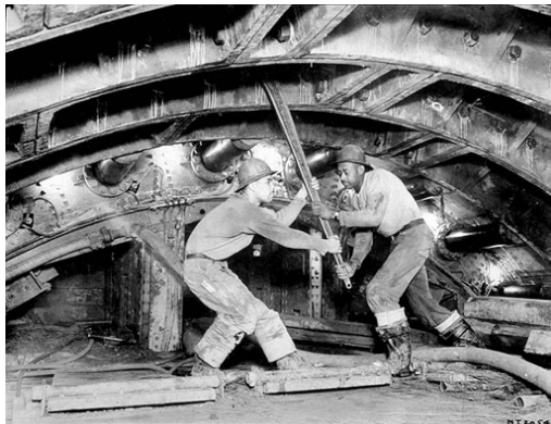
"Sandhogs" wield 60 lb. ratchet wrench to bolt cast iron lining rings in the Queens Midtown Tunnel, February 26, 1939.
