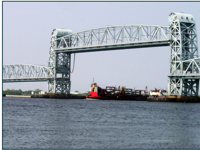
PHOTO CAPTION: Marine Parkway Bridge Vertical Lift Span raised for marine traffic.
