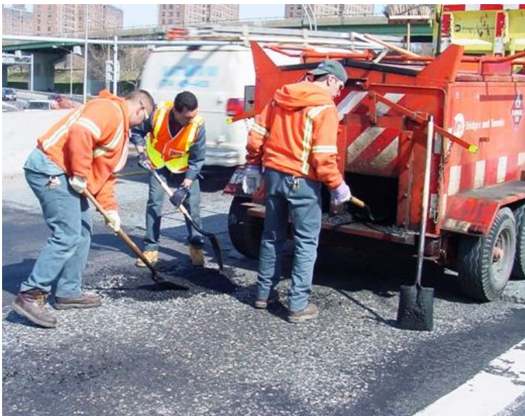
A B&T Hot Box Crew tackles potholes on the Triborough Bridge
