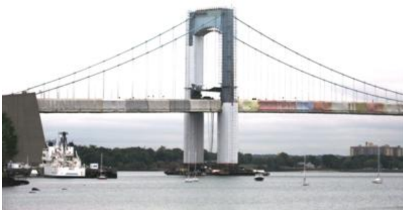
Throgs Neck Bridge shrouded or "encapsulated" in preparation for old paint removal and new painting. All paint removal and application is
