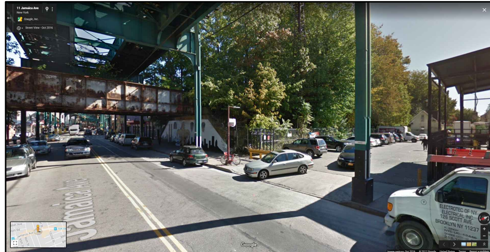
6 WEST SIDE OF TRACKS LOOKING SOUTH EAST JAMAICA AVE
