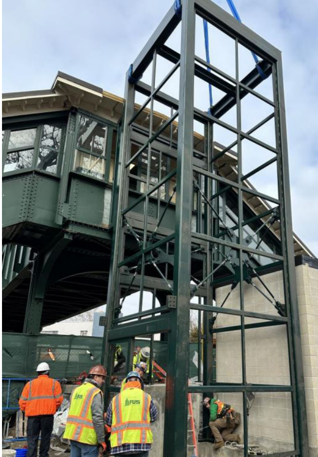
Elevator installation on the Harlem Line
