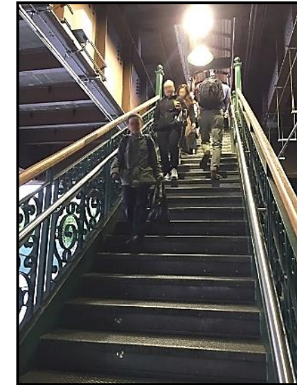
125 th St. Stair Replacement Project (SBMP)
