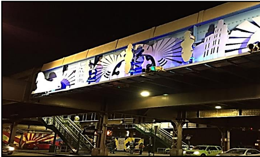
125 th St. Lighting Improvement Project (SBMP)
