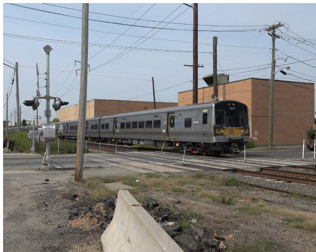
LIRR grade crossing
