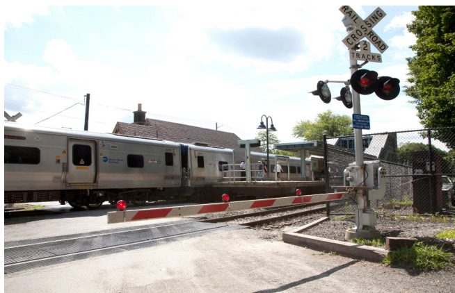
Metro-North grade crossing
