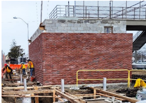
Construction of the new boiler house
