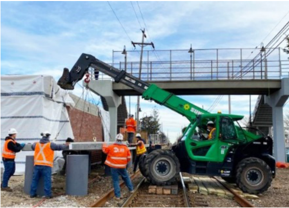
Installation of concrete slabs at Northport Station
