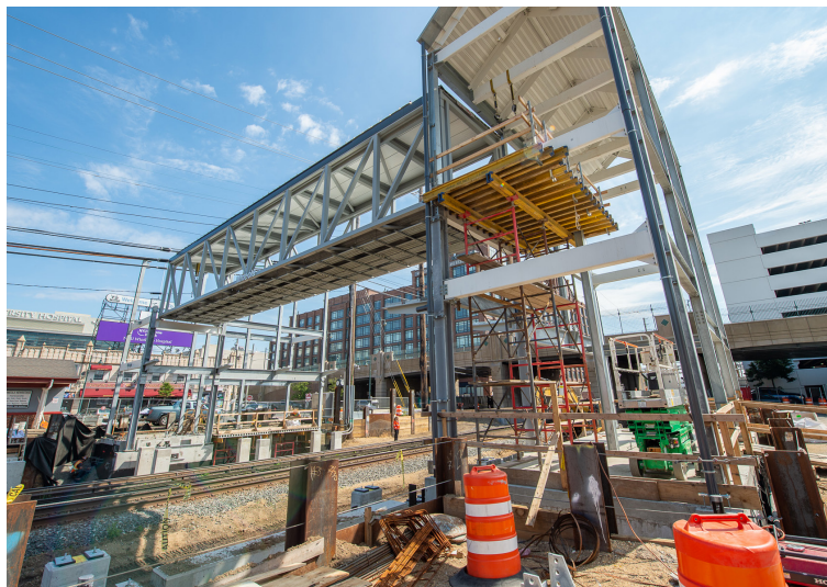
Construction progressing at Mineola Station
