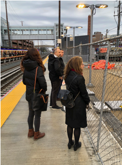
Mineola Mayor Pereira tours the Mineola Station construction progress
