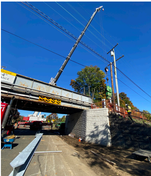
MTA crews work on the Cherry Valley Rd. Bridge
