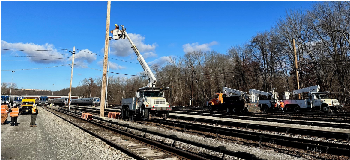
Construction of communications and signal infrastructure along the Harlem Line
