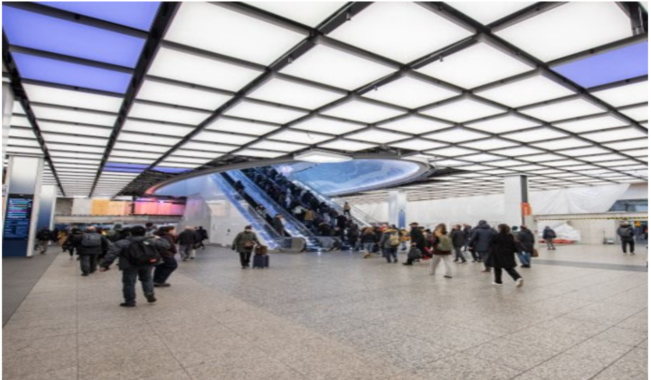
Rehabilitated LIRR Concourse - Widened Corridor and Raised Ceiling
