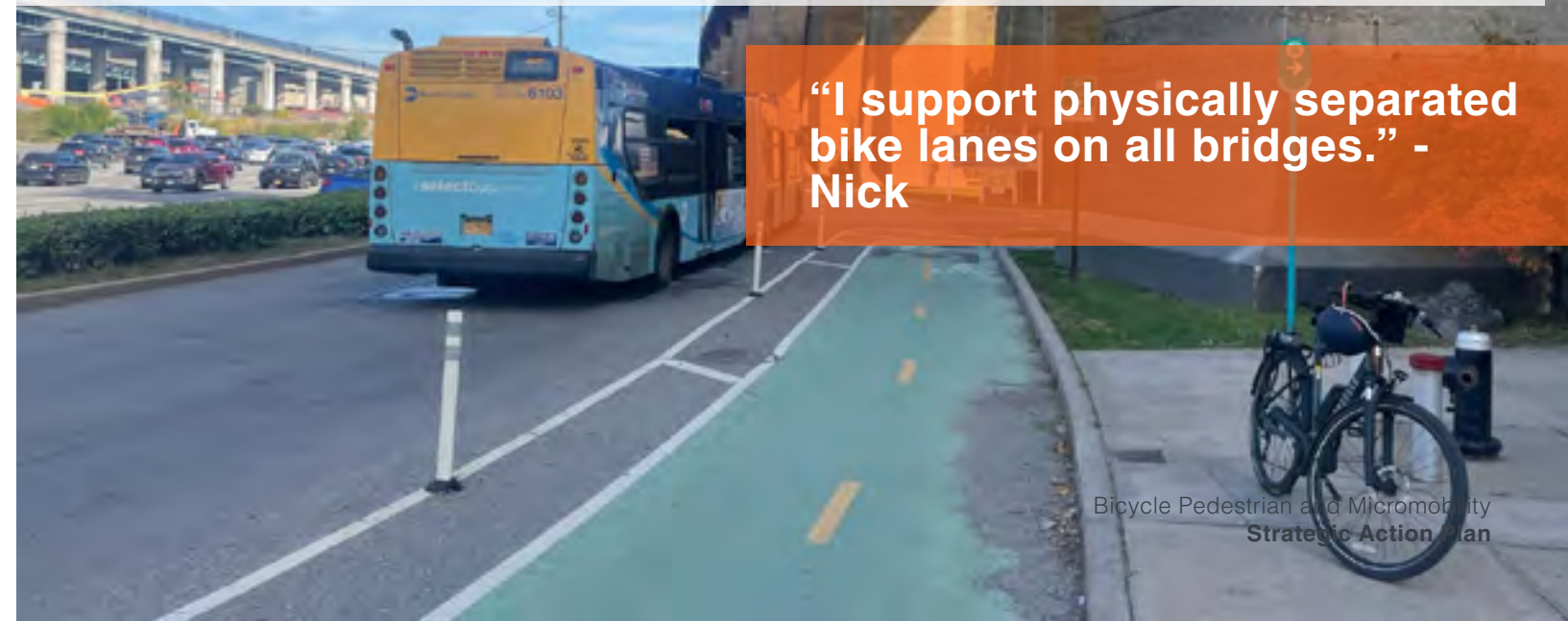
NYC DOT street design on Randall's Island with a protected bidirectional bike lane next to travel lane shared with NYCT Buses. Source: Emily Provonsha/MTA
