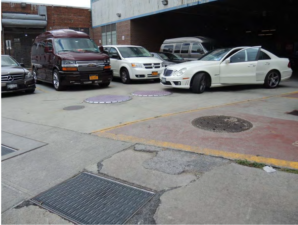
Photograph 9: Lot 46, detail of manholes and grates leading to buried tanks and other subsurface utilities at Tuskegee Airmen Way entrance to Jamaica Bus Depot. View looking southeast from Tuskegee Airmen Way.
