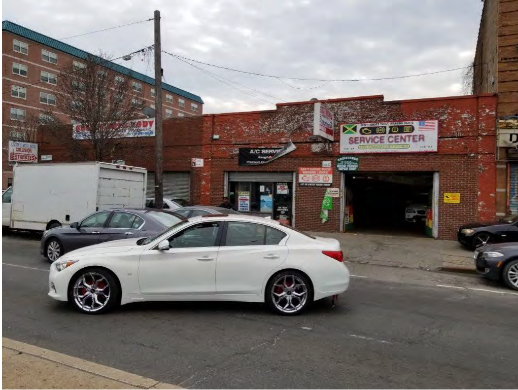
Photograph 21: Lot 90, commercial buildings. View looking southwest from Merrick Boulevard.
