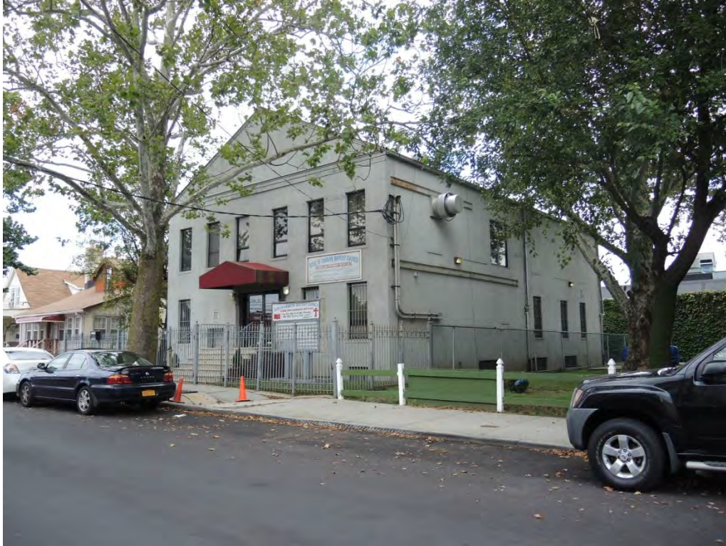
Photograph 27: Present Rose of Sharon Baptist Church (former apartment building) at 104-19 165 th Street. Ivy covered wall in right background marks edge of bus depot lot. View looking north.
