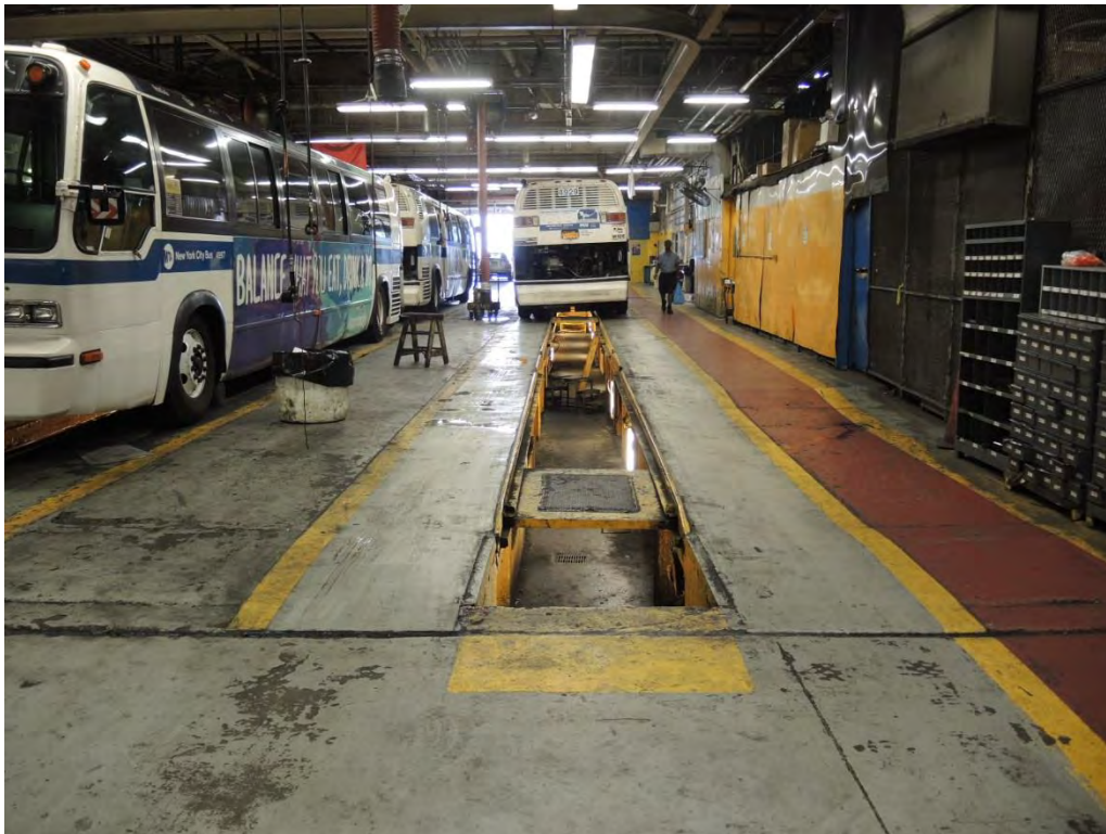
Photograph 10: Lot 46, example of subgrade pit for bus maintenance. View looking northwest.
