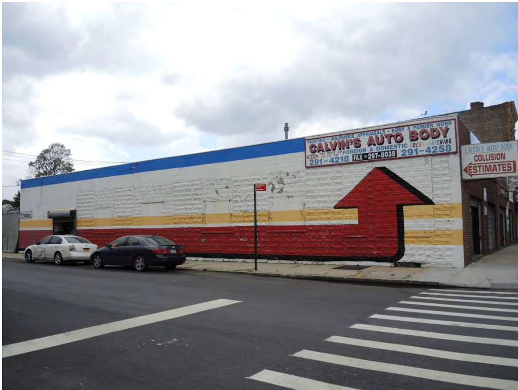
Photograph 22: Lot 90, commercial buildings. View looking northwest from 107 th Avenue.
