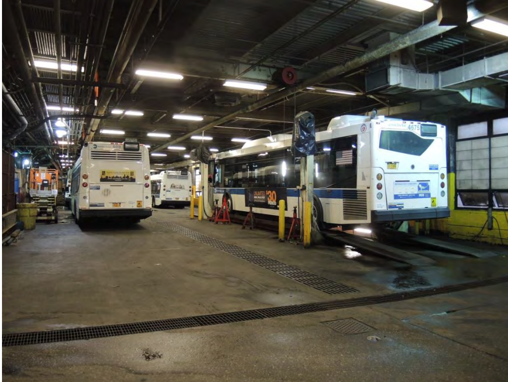
Photograph 7: Lot 46, interior of bus wash area of Jamaica Bus Depot. Note drainage grates in foreground. View looking northwest.
