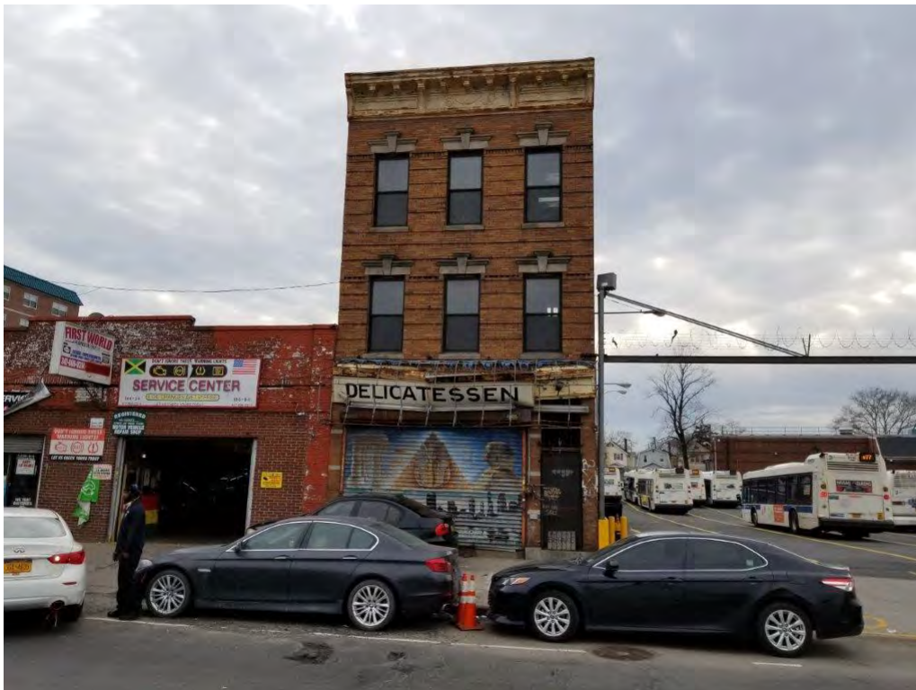
Photograph 20: Lot 89, three-story building. View looking southwest from Merrick Boulevard.
