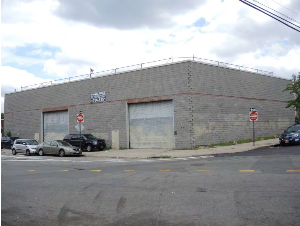
Photograph 1: Lot 41 warehouse building. View looking southeast from Tuskegee Airmen Way.
